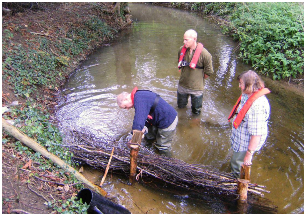
10: Fixing the faggots
