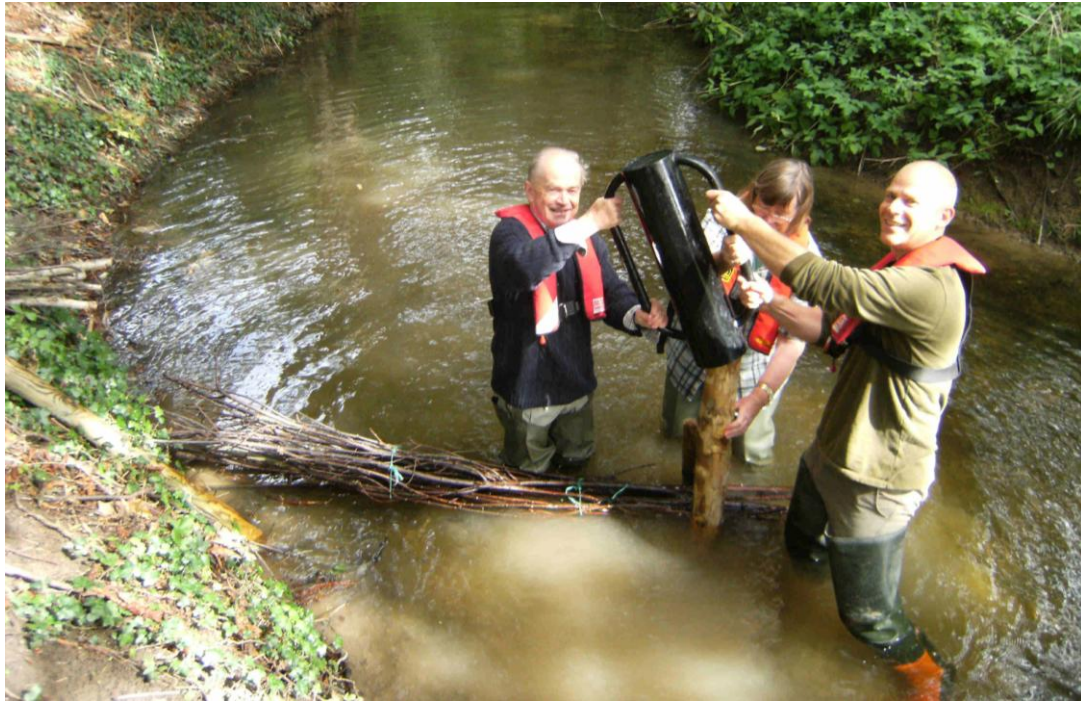
9: Driving the wooden pile supports – Derek and Jennifer
