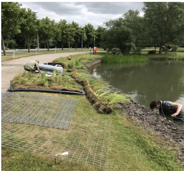
95: Installation of floating islands
