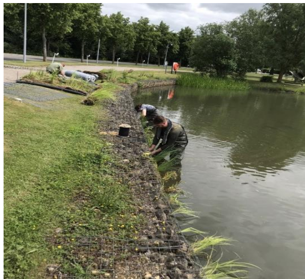
96: Installation of floating islands
