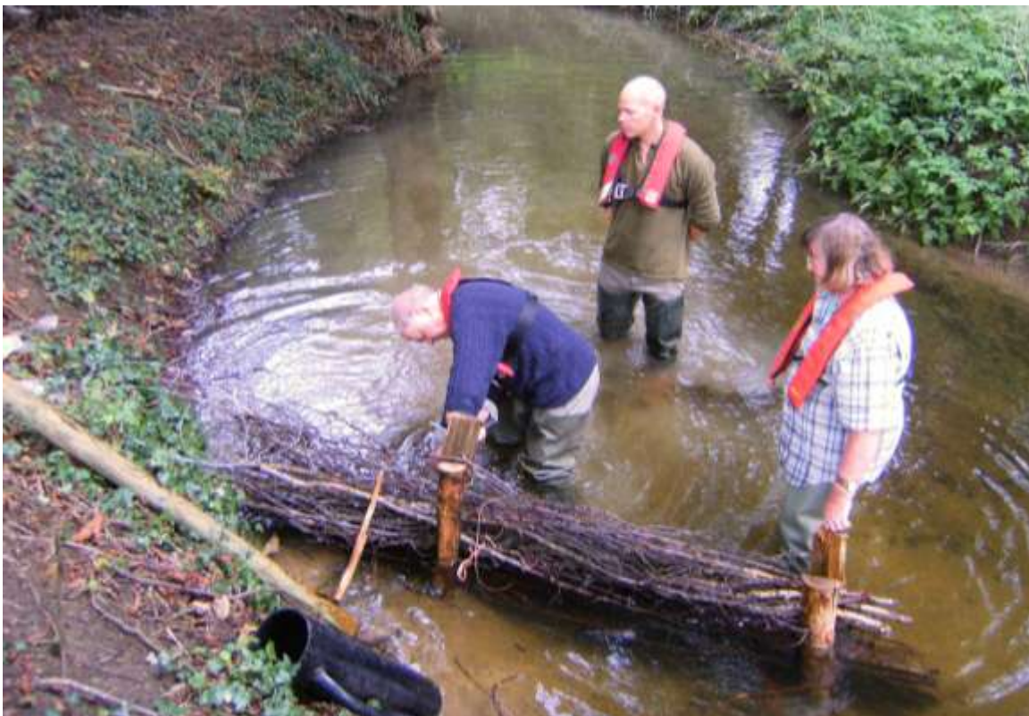
4: Installing Stream deflectors in Sluice Wood
