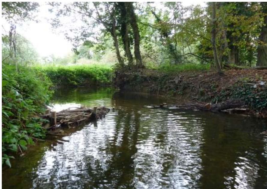
3: Stream Deflectors in Sluice Wood
