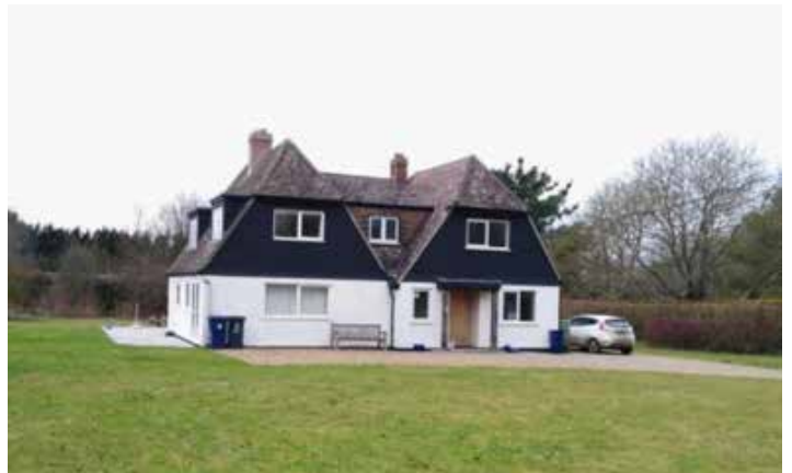
Figure 18: Extended redeveloped South Road property. Roof is sympathetic to original half hipped roof and extended to back therefore restricting extent of frontage facing the road, 2017
