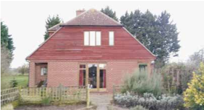
Figure 19: Extended South Road property, keeping the brick on ground floor and wooden panelling on first floor. Half hipped roof style also retained.
