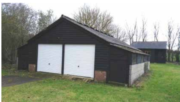
Figure 23: Refurbished piggery on South Road into garage and work shed. Side passages still intact.
